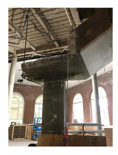
• The existing connector stairwell was completely encased in drywall. Once exposed, it was discovered that the stairwell needs structural repairs and the utilities located in this former chase now need to be re-routed.
